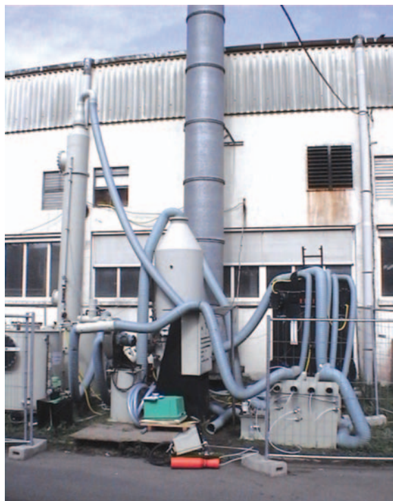
Panel 2: The bio-washer and bio-filter
