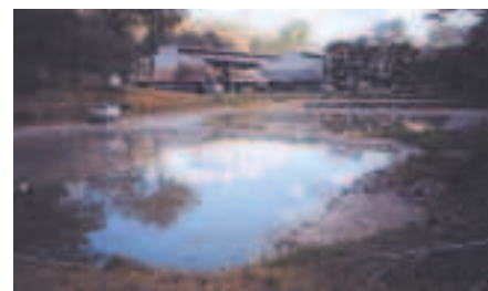
Holding periods of around 10-30 days are used in simple lagooning to reduce the BOD/COD and suspended solids.
