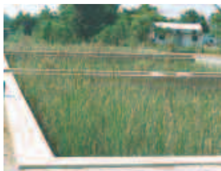
Effluents can be biologically treated by passing them through the root structure of reeds as a cost effective alternative for secondary and tertiary treatment.
