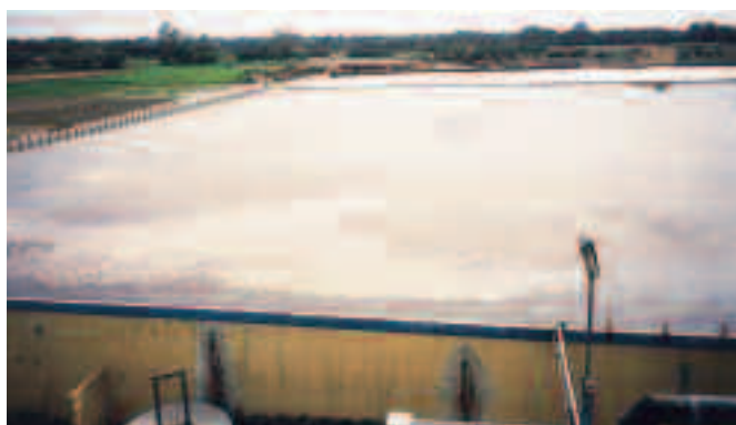
Extended equalisation requires a very large area, as the holding times are long.
