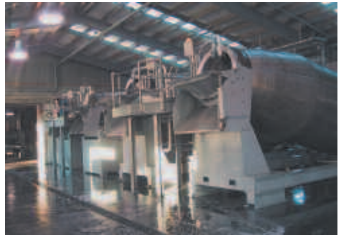
New wet end extension at Tasman Tanning
