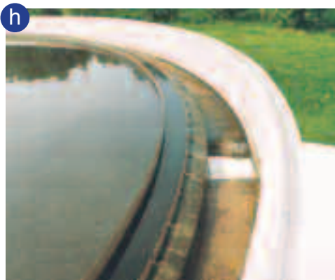
Separation of the very fine bio-flocs as part of secondary clarification.
