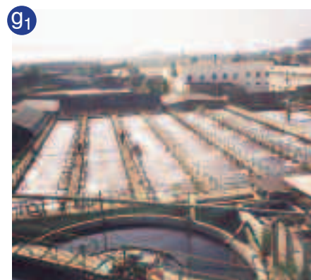
g 1 Activated sludge treatment at a CETP. In this example, aeration is provided by diffused aeration.
