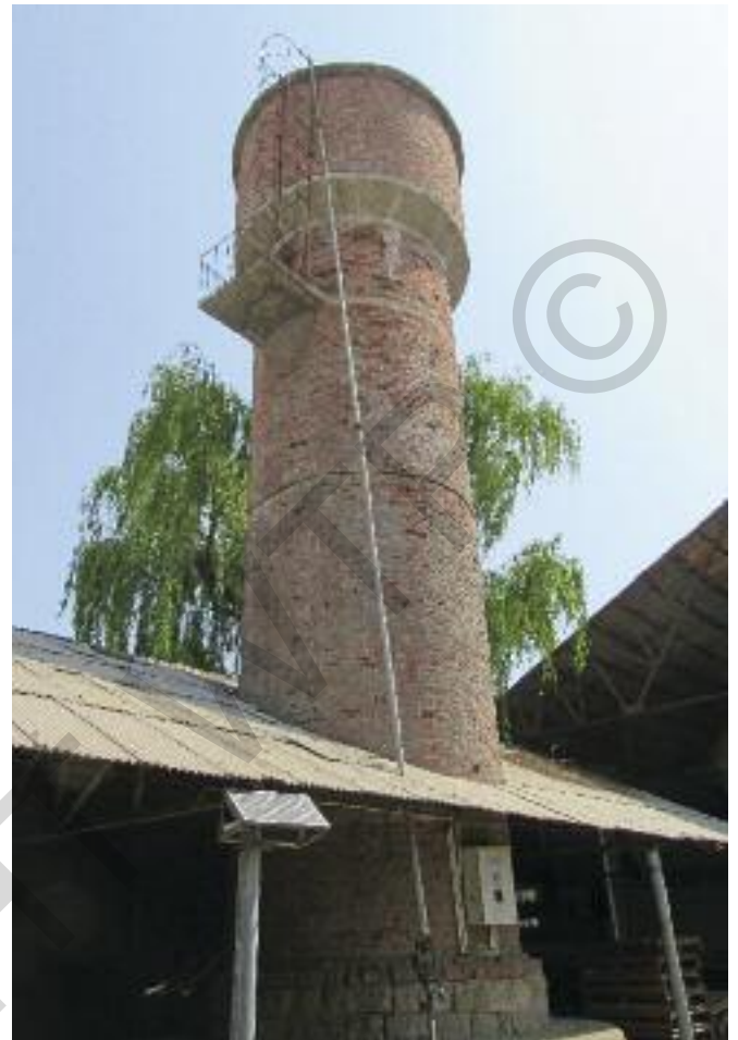
This water-tower, a throwback to the site's former existence as a brickyard, is still in use. It stores water for use in the dry months.
