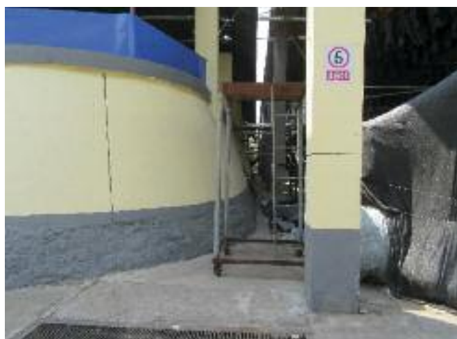
The original brick kiln has been redesigned to be used as a drying chamber. Being approximately 20 metres wide and 50 metres long, the top of the kiln acts as a storage area but also houses the vacuum dryer condenser where the extracted moisture from the drying operation is reused.
