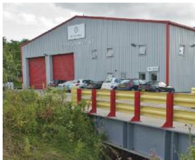
UK-based Bridge of Weir Leather Company operates its own on-site thermal energy plant, to which it sends much of its solid waste.
