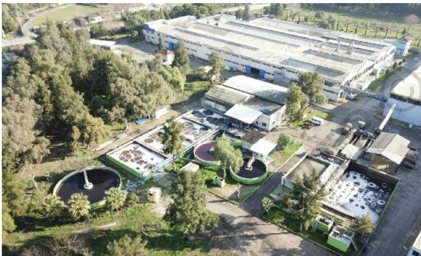
The effluent treatment plant at Torbali.
