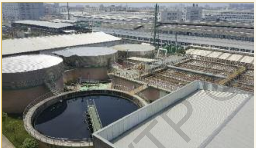
The common effluent treatment plant at Andong, used by Xingye and a number of other leather manufacturers at this new cluster near Jinjiang. In 2011, there was almost nothing here.
