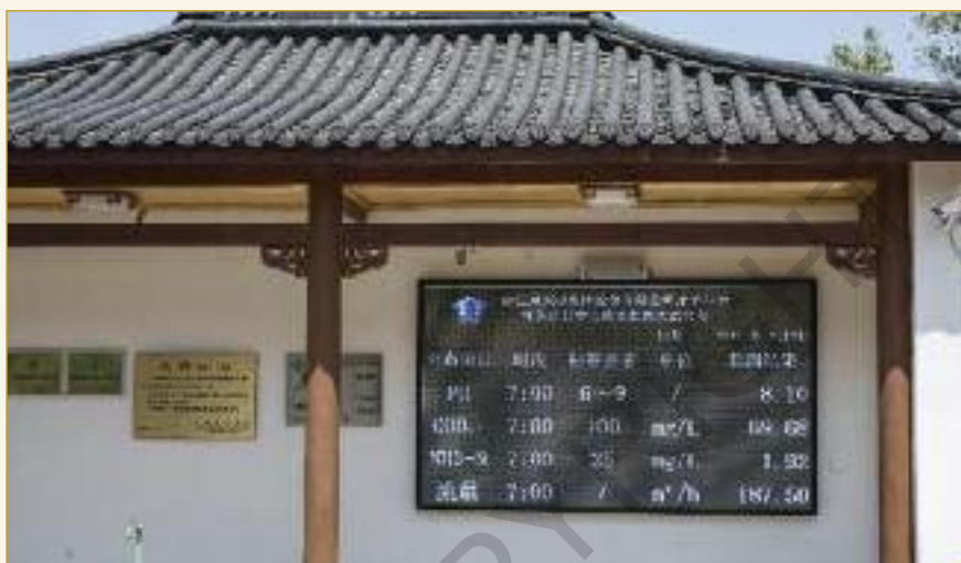
Water flows from the tannery straight into the important Qiantang river system. Zhejiang's provincial government carries out 24-hour remote monitoring of BOD, COD and ammonia.
