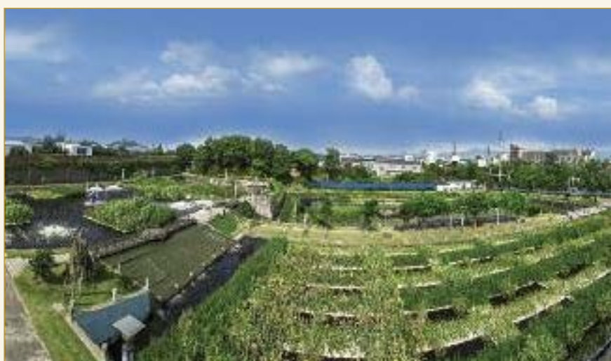
Part park, part effluent treatment plant, the TTX wastewater facility is an attractive place.
