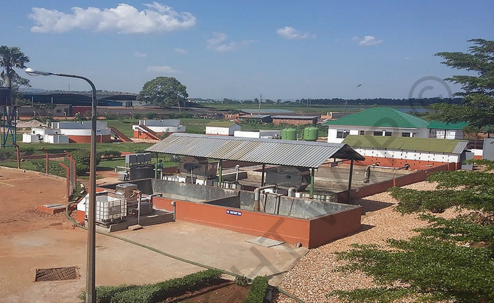
LIU's effluent treatment plant.
