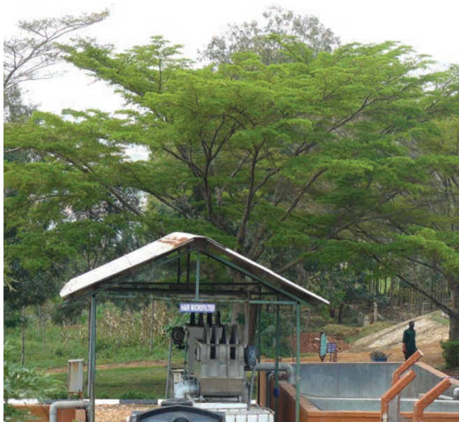
Just visible through the trees, the tannery is located less than 200 metres from the precious and vulnerable resource that is Lake Victoria.
