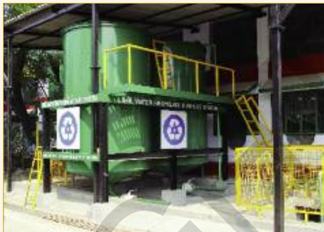
A recovery system for collection and reuse of used unhairing/lime floats is in the final stages of construction. The discharged floats and the recovered supernatant will be held in storage sumps constructed below the assembly.
