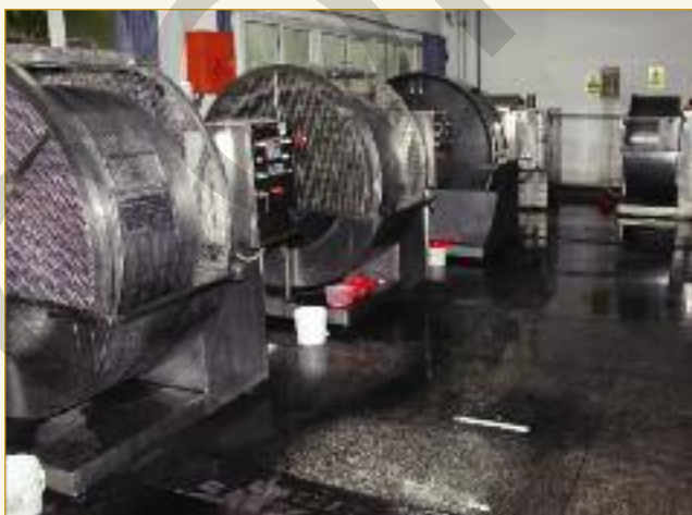
Shows part of the pilot plant for small-scale development work comprising seven stainless steel drums of various sizes. Physical and chemical testing laboratories are located nearby.
