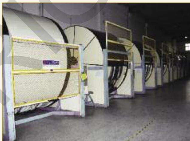
There are 17 milling drums in total, set in two banks.
