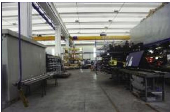
Section of new Feltre Works where Emmezeta machines are also erected. Toggle dryer O1ne is seen in the background being assembled.
