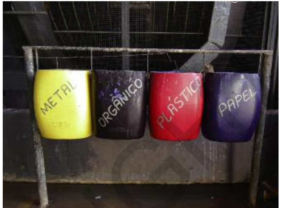
Sets of these rack mounted and colour-coded recycling containers are used extensively throughout the plant, before delivery of the waste to the final segregated area.
