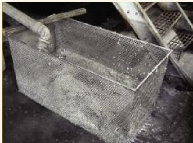
As a first stage of effluent treatment, all of the pre-tanning floats from the fish skin production are coarse screened on discharge from the drums to remove fish scales using easily moved stainless steel perforated baskets.
