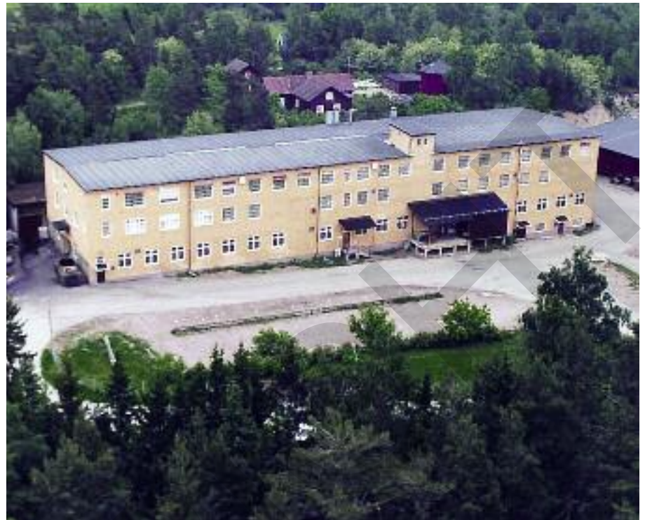
The tannery is set in a heavily wooded area, and next to a small lake. On two sides of the tannery there is housing for local residents, but also housing for second homes for holiday purposes.
