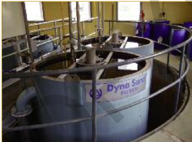
The effluent is fully treated by an external provider at 1.5 km from the tannery. The tannery effluent, after full primary and secondary dosing is mixed with treated domestic effluent. Tertiary treatment comprises chemical dosing and clarification, then filtration through this pair of sand filters.
