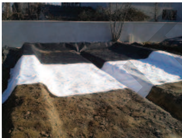
Panel 2: Construction of the remediation site.
