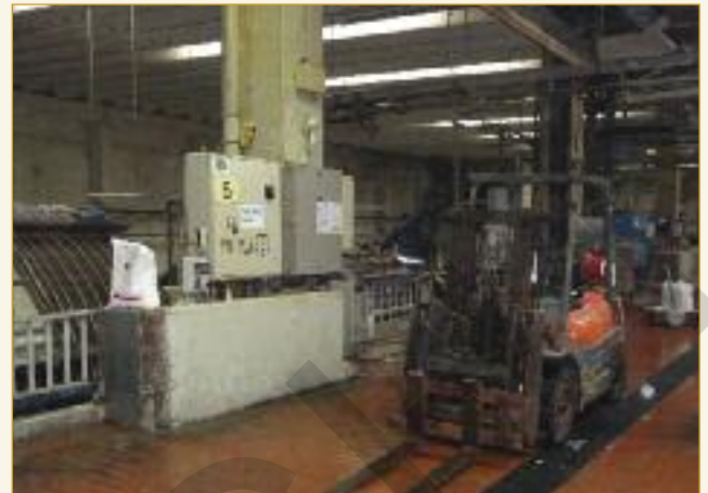
The tiled floor of the mezzanine with central drainage ensures that the whole service area can be readily washed to maintain the highest standards.
