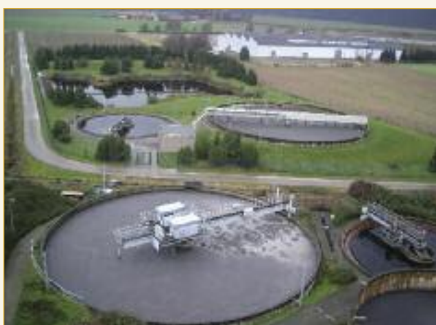
After final clarification the treated effluent is discharged into a natural pond (top left). The outflow from this pond runs into a drainage ditch before final discharge into the nearby river.
