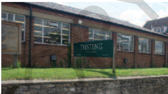
Manufacturing wing of the Warehouse at Lavendon. CREDIT: WTP
