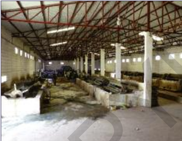
Shows the clean and spacious interior for the soaking, unhairing and liming section of the tannery.
