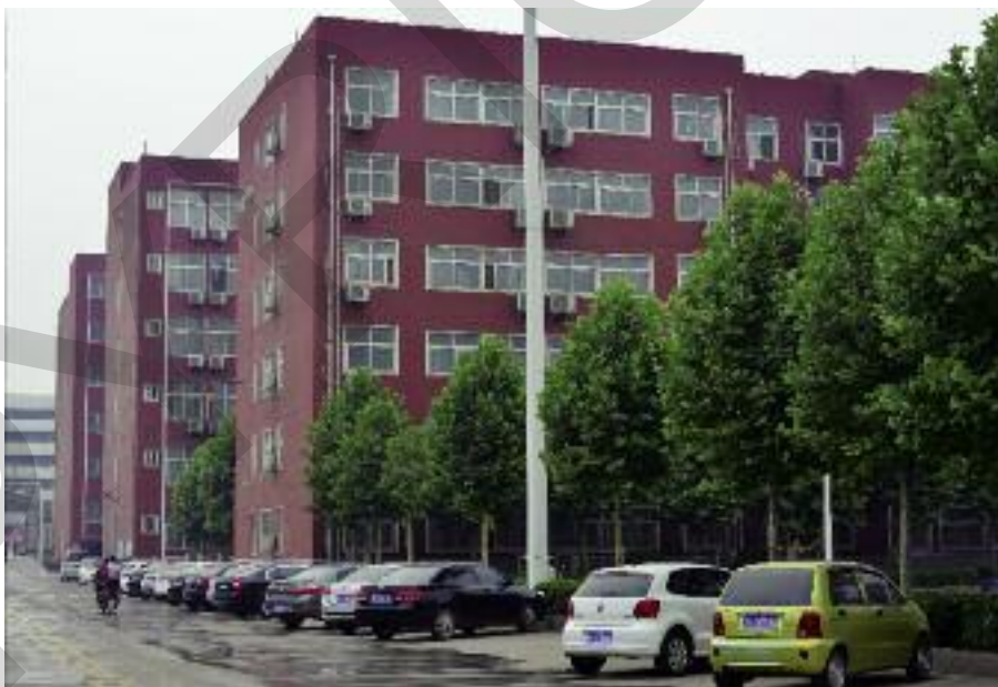
This image shows part of the accommodation built for the workforce at Henan Prosper. It is often the case that over and above husband and wife who work on site, children and grandparents also are housed here.
