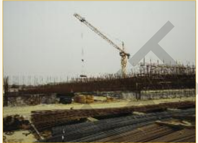
Work has commenced on a new effluent treatment plant that is capable of treating 40,000m 3 /day. This will replace the existing systems, ensure a very high level of performance to meet pending legislation, and allow for considerable future expansion.
