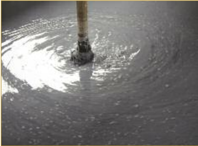
The separation and treatment of chrome-containing wastewaters is a key component in effluent treatment. This shows the mixing and precipitation of chromium salts using sodium hydroxide before separation and dewatering of the precipitates using a filter press.
