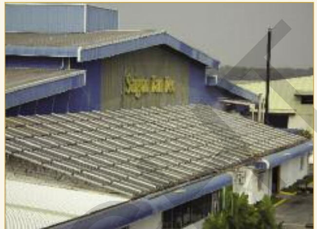
Solar energy is being used for provision of hot water. Three large holding tanks are used, with the cooler water drawn from the base of each tank for heating and recirculation. This provides water at 75°C, although it can be assisted if required.
