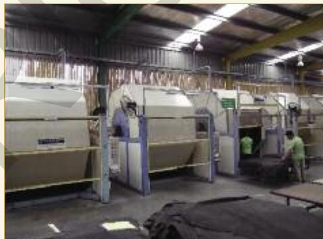
Bamboo is used in the place of solid walls in parts of the building. This ensures a gentle flow of air throughout the plant, but also provides natural lighting in the immediate work areas.
