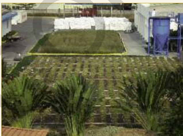
Two of the reed beds used for polishing treatment. The reeds in the bed in the foreground have just been cut having reached a height of about 2.5 m. When dried and chipped these will be added to the biomass boiler.
