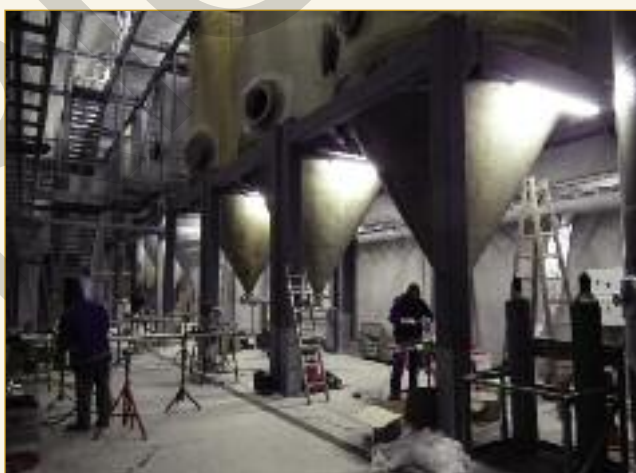
This shows the conical base of six settling vessels being installed for the recovery of proteins following the acid precipitation of unhairing/liming wastewaters and washings after sulfide removal. The objective is to reduce the impact on the biological plant, and to recover solids with secondary use to avoid disposal.
