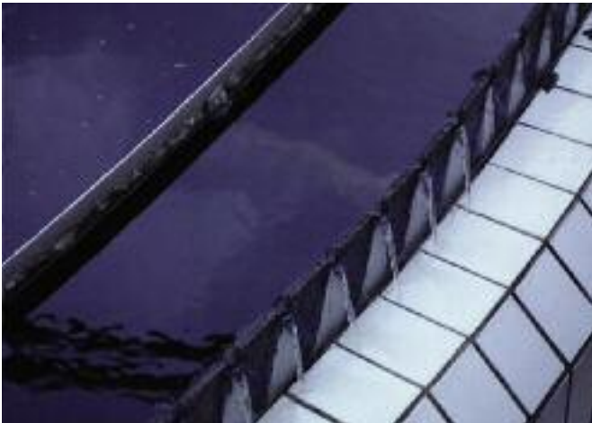
Effluent following secondary clarification, before flotation and filtration using activated carbon. The quality is particularly high as the discharges are into the adjacent river; this receives effluents from other manufacturing operations, and eventually flows over the border from Austria into Hungary.
