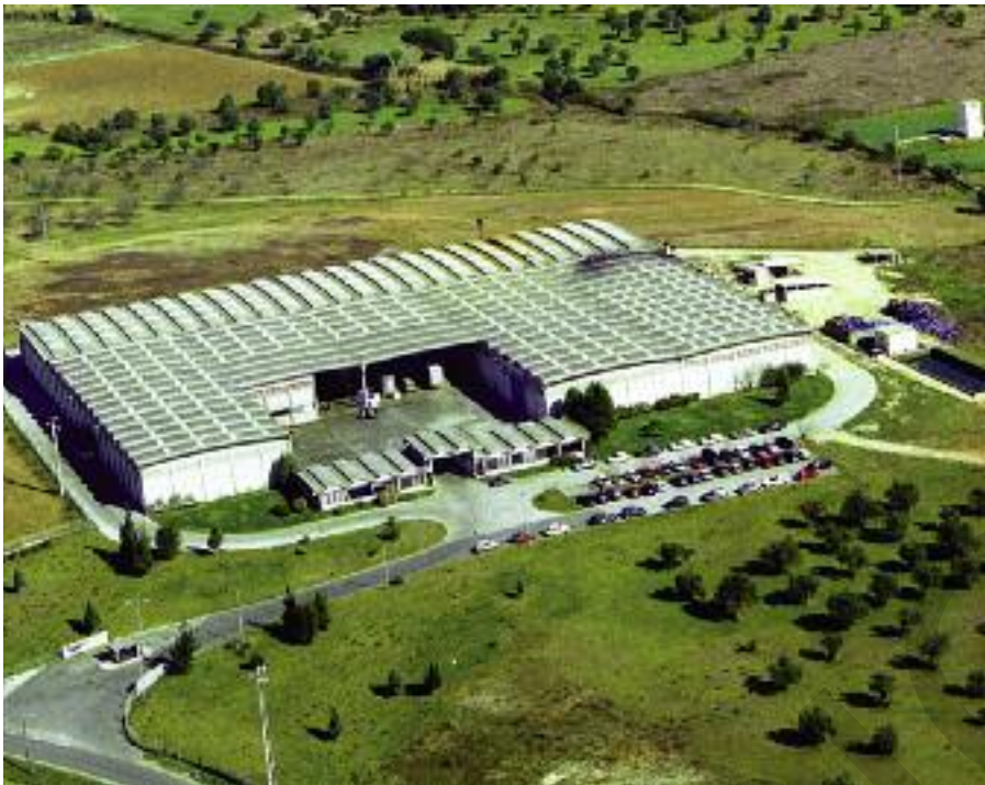
The land around the site of the tannery is naturally contoured and lends itself to landscaping as shown in this image of the entrance to the tannery.
