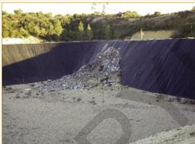
Solids from the effluent treatment plant and general solid waste from the tanneries are stored in separate encapsulated landfill sites adjacent the CETP. The surrounding area is being planted with trees.
