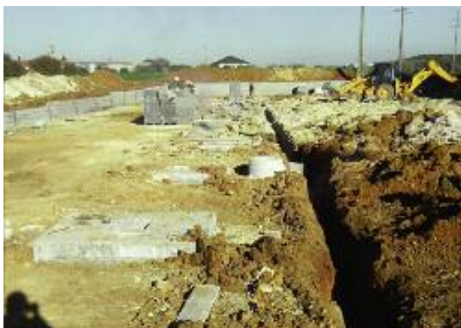
The tannery is being expanded into a new wet end facility adjoining the existing buildings. The trench is part of the construction of the drainage arrangements for separation and recycling of wastewaters from wet processing and machine operations. The building will be prefabricated with a construction deadline of early 2014.
