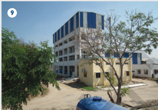
The whole recovery plant is housed within the blue and white building. The five story part accommodates the seven evaporator units.
