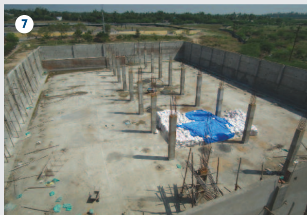
An additional storage facility is under construction for secure storage of the recovered salt. Investigations are taking place to find a use for this impure product.
