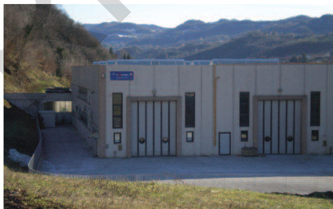
The new plant at Chiampo, a few miles north of Arzignano in Vicenza Province.
