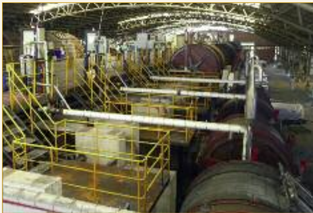
Part of the dyeing department, and the materials weighing and dispensing area that services drums set on both sides of the mezzanine.
