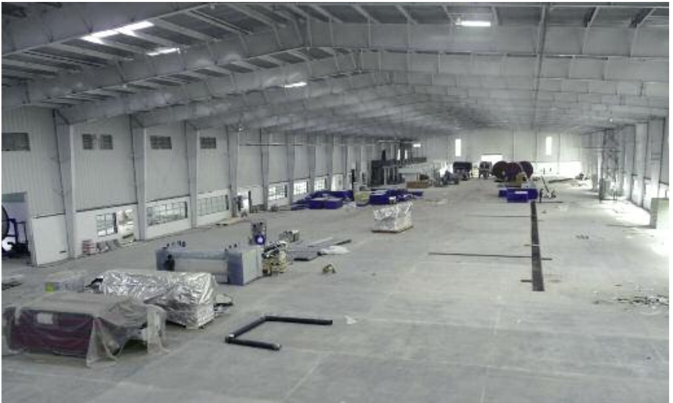
The first drums are being installed in the new tannery for the manufacture of athletic and upholstery leathers.
