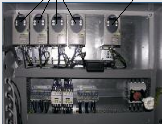
Inverter Controls of Airflow
