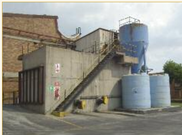
This plant is designed to receive used lime liquors and washings. After grease and solids removal, the recovered liquors can be preheated then, together with chemical adjustments, used as the liming/unhairing floats.
