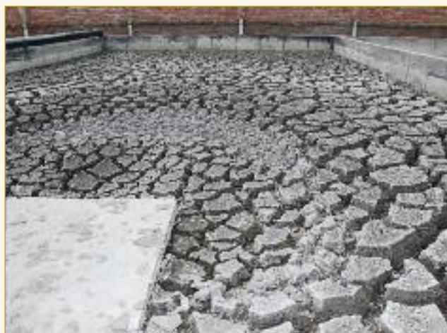
Sludge-drying beds work well in temperatures that can reach 48°C.
