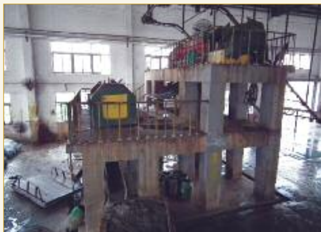
This shows the arrangement of the three pairs of fleshing machines. Half of the hide is fleshed on the upper machine, with chute feed to the lower machine to complete the operation. The hides are delivered to floor level, then stacked (onto a pallet set at an angle). The fleshings are delivered into an open container.
