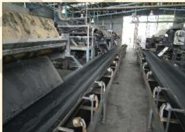
At the León CEPT, belt presses are used to dewater the sludges following tannery effluent treatment. Chrome containing sludges are securely deposited on site, but biological sludges are further processed to generate methane.
