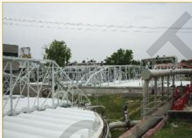
Air ducted from the encapsulated homogenation tanks is treated to oxidise hydrogen sulfide gas and produce colloidal sulfur in the following manner:
