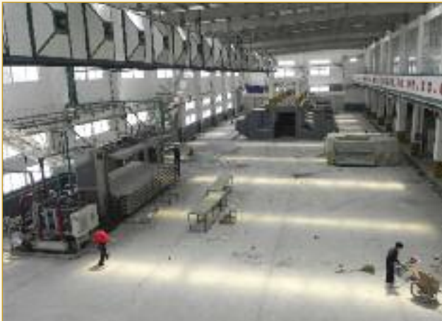
The new wet blue to crust department. Top centre shows the plinths for supporting the two rows of dyeing drums, and structure for the feed mezzanine.
