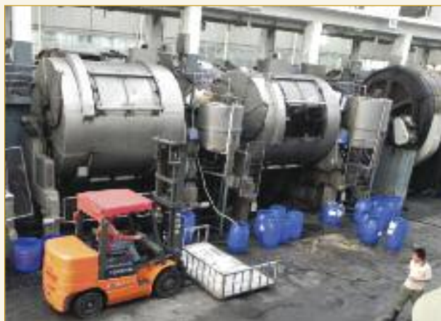
Part of the dyeing department. There are five stainless steel tri-compartmental dyeing vessels, and ten 3.0 x 3.0 m 2 wooden dyeing drums in this department.
