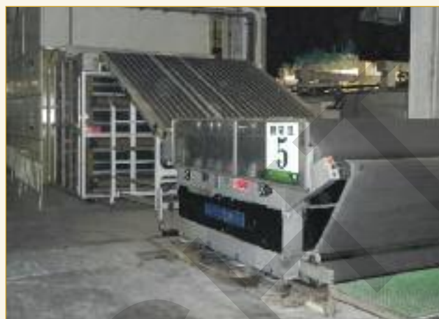
One of the two Cartigliano wet stretching (wet staking) machines with feed to high speed drying and conditioning units.
