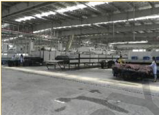
Two spraying lines have just commenced operation. A roller coating machine is currently being installed for the centre unit.
