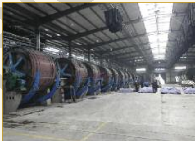
Part of the tanning department. Once the installation of the tanning drums and services is complete, 52 drums will be in use.
