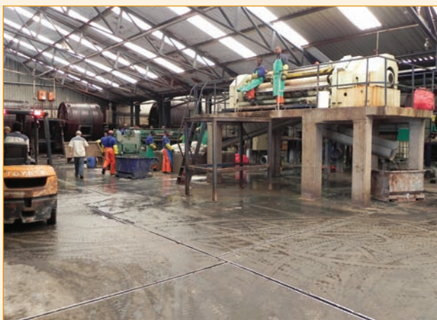
General view of the beamhouse. The processing vessels are of various sizes and configurations to suit sheepskins, bovine hides and exotic skins.
