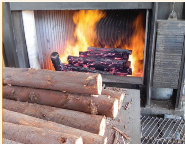
Logs from renewable resources are cut to length and loaded onto a conveyor. As fuel is needed, the furnace doors open, and the logs automatically feed onto the fire bed.
