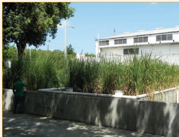
Reed beds are under evaluation for secondary effluent treatment to reduce the COD, and if successful, land is available for a full scale plant. A reduction in COD load from the present maximum level would in turn enable an increase in production.
