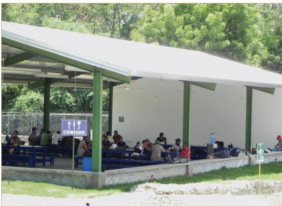
This open-air eating facility for the workforce, fairly near the plant, has just been completed.
