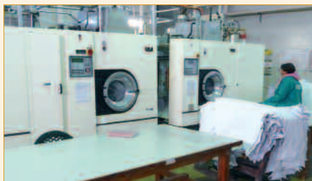
Industrial dry cleaning unit to ensure full grease removal.
