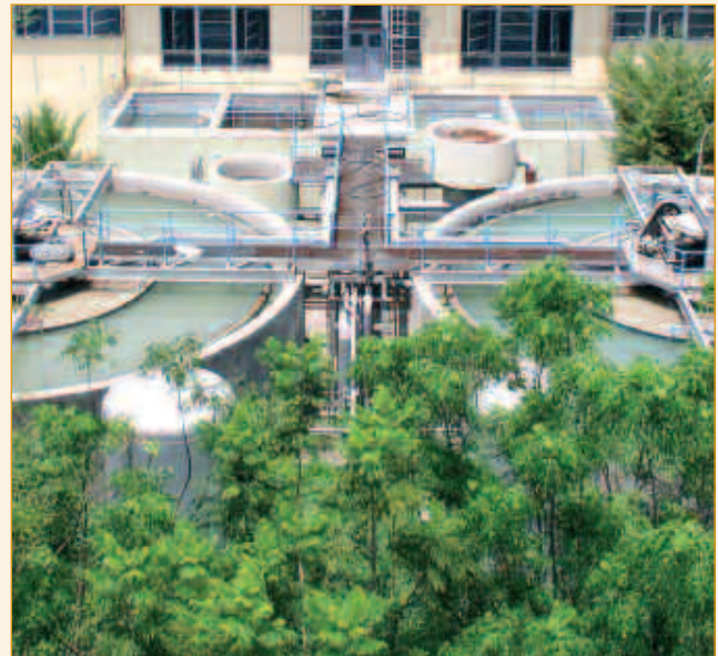
This water treatment plant will soon be converted for use as cooled water holding tanks.
