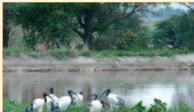
Part of the lagoon effluent treatment system.
