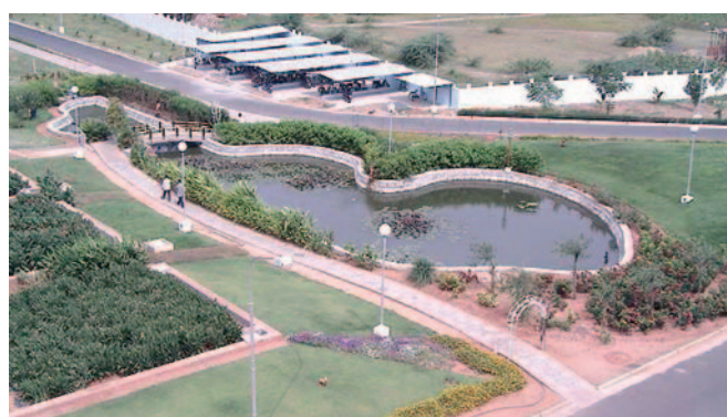
The reedbed at the Aravind Eye Hospital, Pondichery, Tamil Nadu, India, has a capacity of 540 m 3 /day. The untreated effluent has a BOD of around 100 mg/l and treatment achieves an outlet with a BOD less than 10 mg/l.
